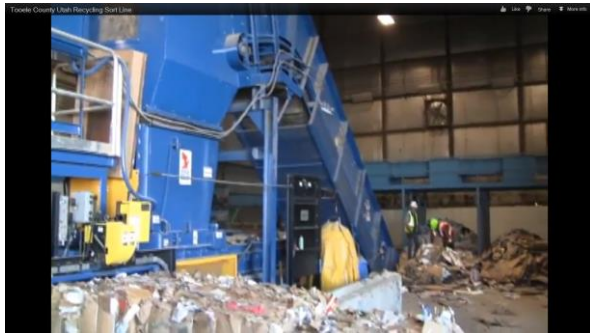
RECYCLING FACILITY -Bailer
